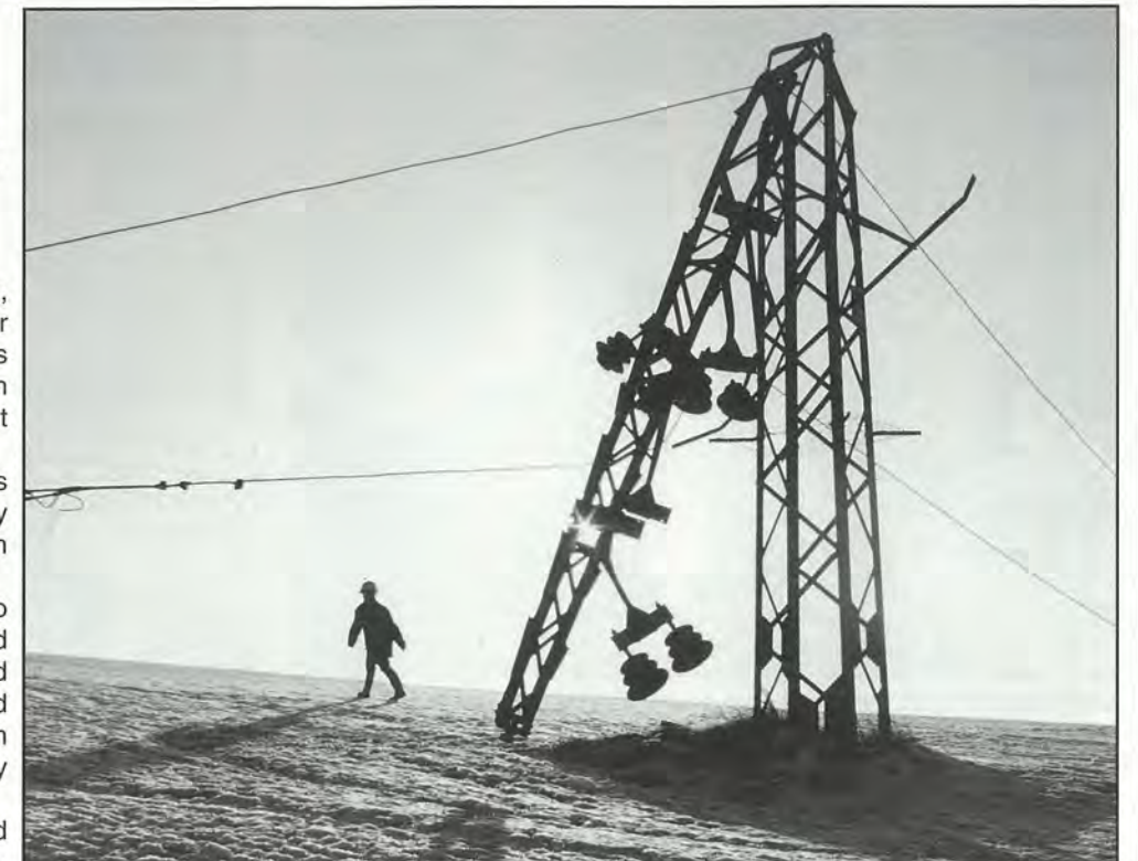
A steel tower snapped in half during the severe weather in Scotland.
